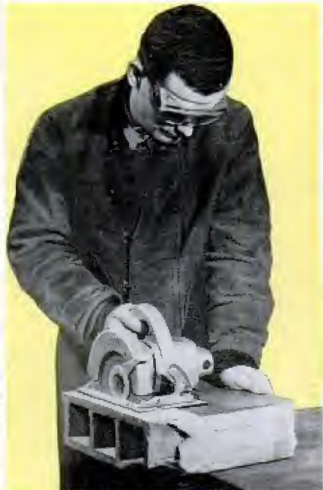
Above, note similarity of operations of cutting wood and clay tile. Saw is held in same manner. Woodcutting blade is replaced by abrasive disk for cutting tile. Right and below, saw squares up broken pieces of hollow tile and concrete for re-use
